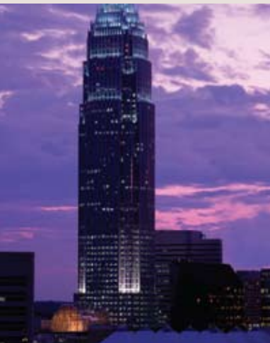
Pressure Interceptor used in high-rise building – Charlotte, NC
